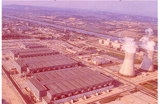
View of the Georges Besse enrichment plant of Eurodif
